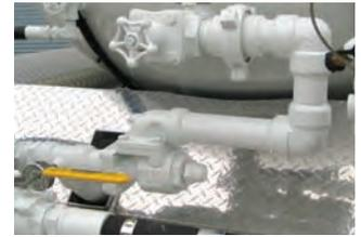
Blackmer differential bypass valves are designed to protect pumps and system components from excessive pressure damage, and no CO<sub>2</sub> pump installation is complete without one. Blackmer offers five different models that provide full-flow pressure control to 250 U.S. gpm (946 L/min.) at 120 psid (8.27 bar). Installation is easy with NPT tapped ports in sizes from 3/4 in. to 2 in.
